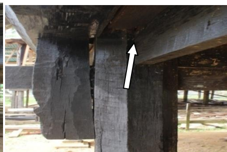
Figure 4. Sigitan (Energy-efficient green architect)
